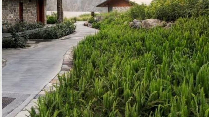
ROAD OVERALL ( MIX STONE EDGE & CONCRETE BRUSH FINISH/BITUMIN BLACK TOP)
